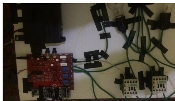
Figure 4 Experimental setup using the electronic card designed for the sprinkler irrigation system
