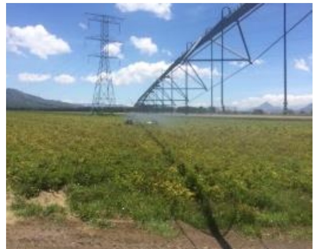
Figure 6 Bypass of secondary piping to the sprinklers operated with the use of the electronic card
