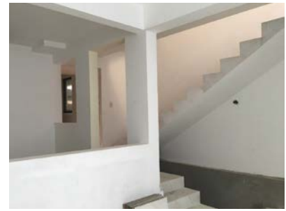
Figure 4: Walls and ceilings covered with gypsum plaster.
